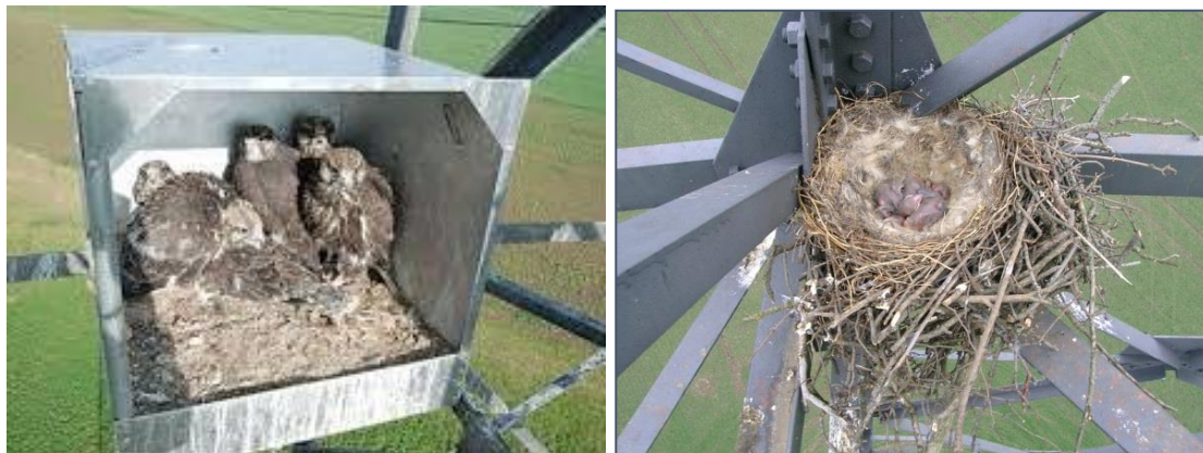
Figure 5-4: Nesting box installed on power line pylon and natural nest
