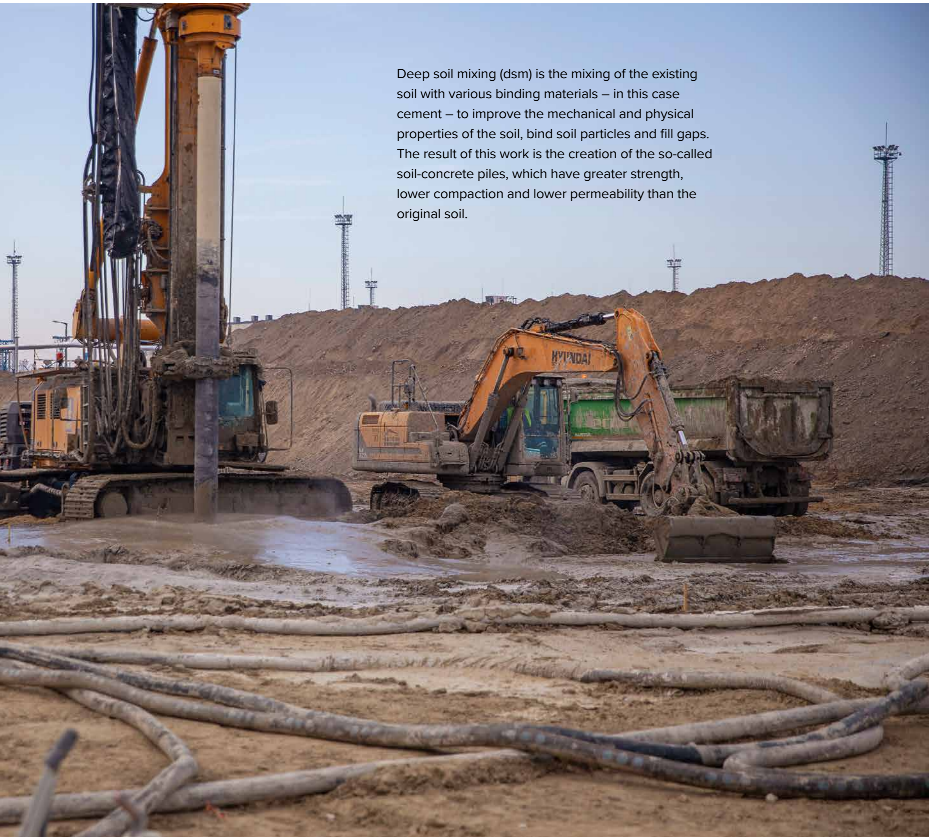
The soil improvement is carried out by Bauer's BG 45 machines with a power of 433 kW.
