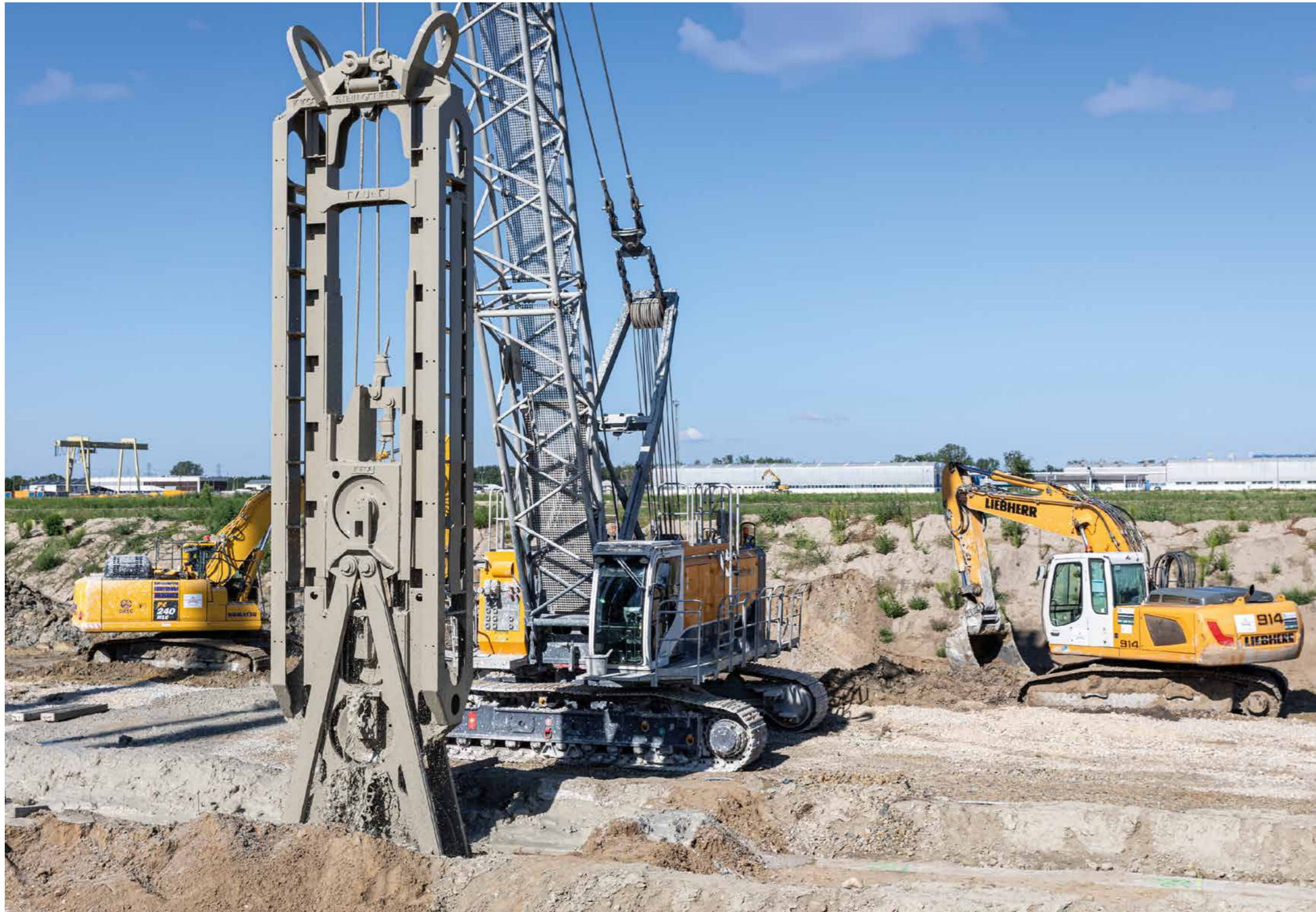
The construction of the cut-off wall was carried out by Bauer's MC 76, 99-tonne, high-capacity, self-propelled, crawler-type machines.
